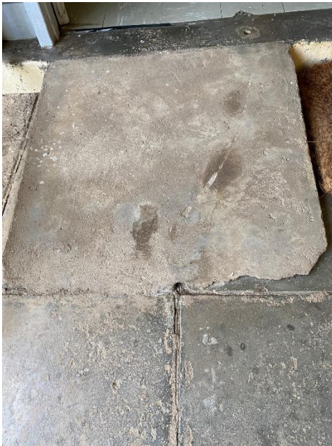
Accessible ramp however, it has no handrails.
